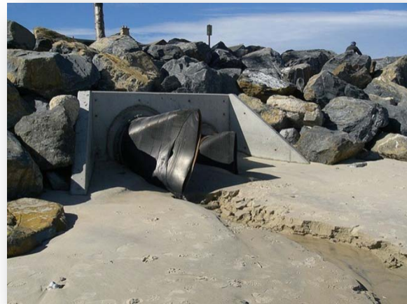
Figure 2: One Way Flow Valve
