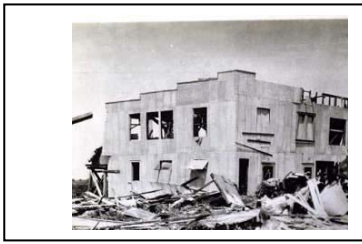
1928 Storm Damage - WPB
