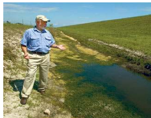
Evidence of Internal Piping
